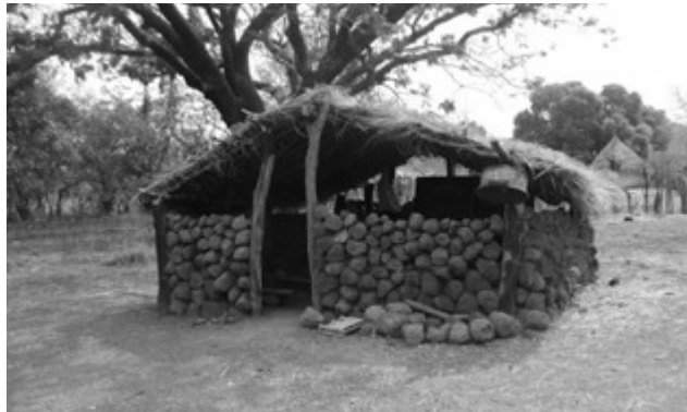
Village school in Djirne: In recent times, a number of new schools and even some universities have been established in order to at least meet the quantitative targets of the Millennium Development Goals by 2015. | Source: © KAS Senegal/Mali.
