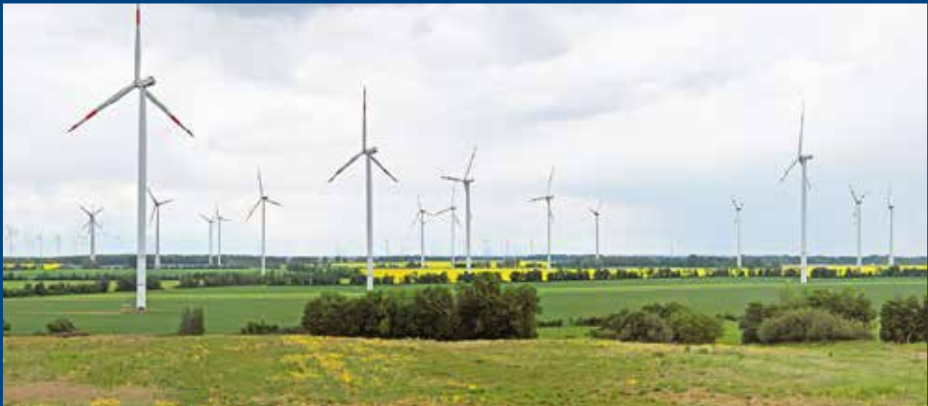
In the federal state of Brandenburg, wind power was rapidly expanded owing to annual grants of several million euros. Source: © senorcampesino, iStockPhoto
