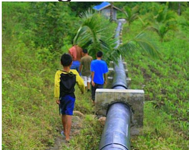
HYDROELECTRIC PLANT --- Children walk along modular tubes where water from a river in Buldon, Shariff Kabunsuan flow down to a paddle wheel attached to a turbine generator now supplying electricity to more than a hundred houses in the area.[]
