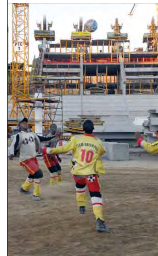
A football game held during the construction of Cape Town Stadium, South Africa. The construction was monitored by an environmental control officer. (Source: Bruce Sutherland, City of Cape Town)
