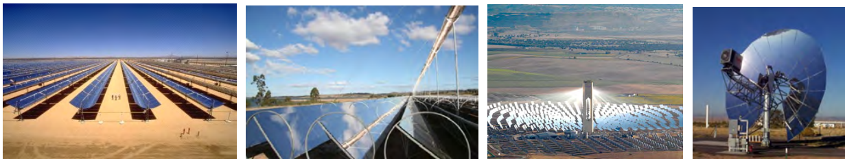
Figure 49: From left to right: solar parabolic trough system [4.33a], Fresnel system [4.33b], power tower [4.33c], and a parabolic dish system [4.33d]
