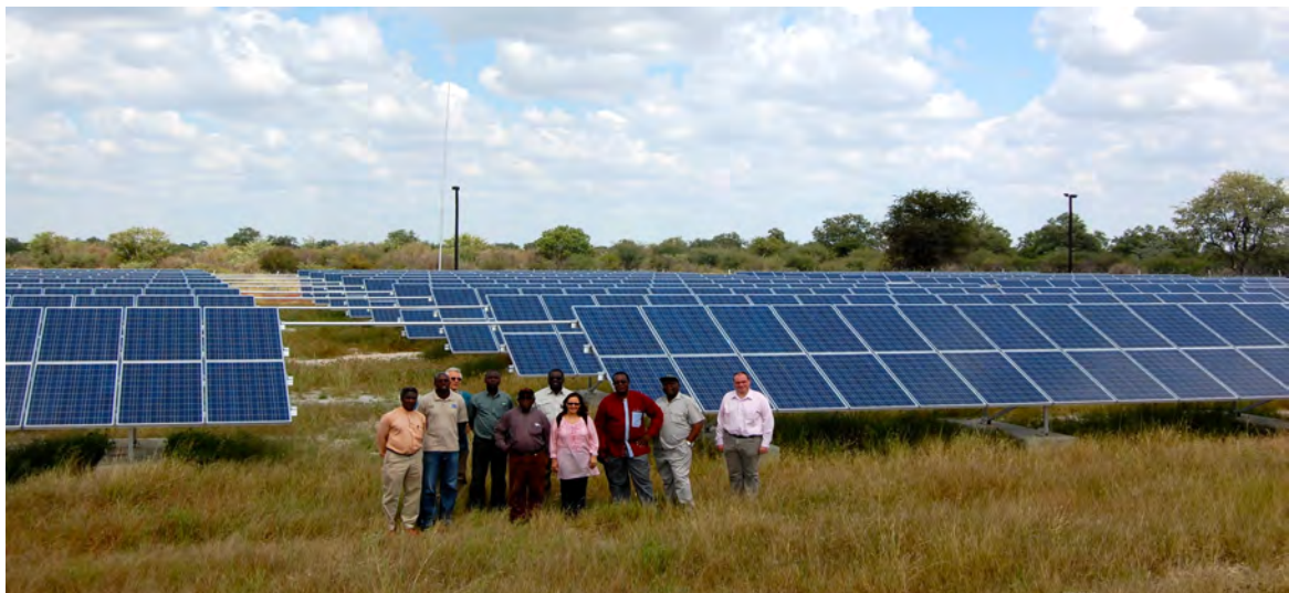
Figure 40: Solar PV array of Namibia's largest solar-diesel hybrid system at Tsumkwe [4.14]
