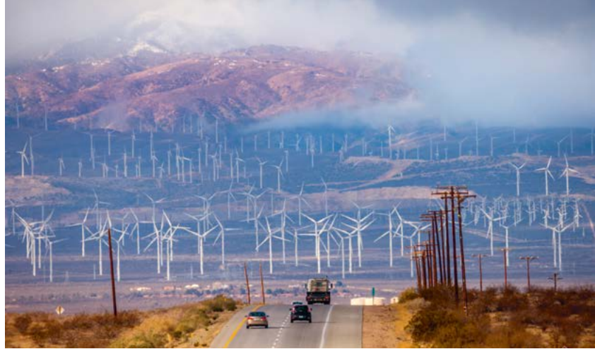
With around 5,000 wind turbines, the Alta Wind Energy Center in Bakersfield is one of the largest wind farms in the world. Source: © Spondylolithesis, iStockPhoto
