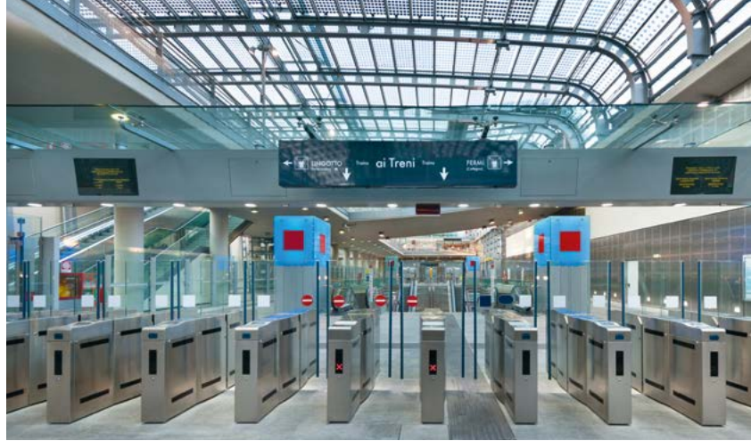
The glazing of the railway station Porta Susa Torino is equipped with mono-crystalline photovoltaic cells. Besides generating electricity, they also act as a sun shield. Source: © Dario Egidi, iStockPhoto
