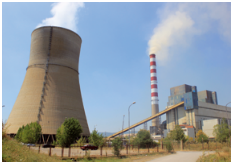
A lignite-fired power plant near Obilić. Kosovo wants renewable energies to cover 26 percent of its energy needs by 2020. At the moment they account for less than 3 percent.
