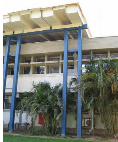
The classrooms are now being protected by special steel constructions
