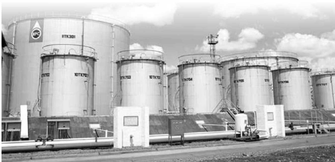
The refinery at the Kenya Pipeline Company.
