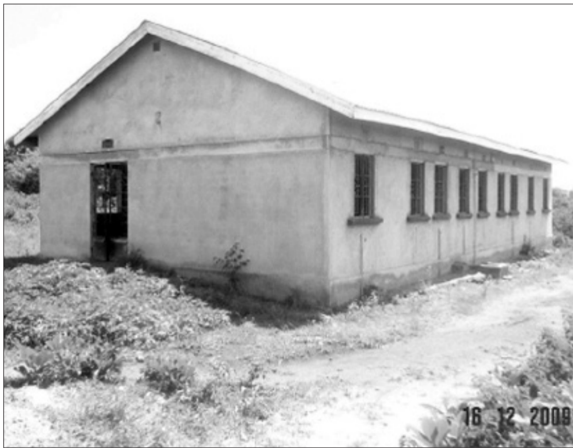
Stalled Burumba Dispensary which has purportedly spent a total of Ksh1.8 million. The former local project development committee has been replaced for allegedly failing to exercise transparency and accountability. Photo/Nyakwar Odawo
