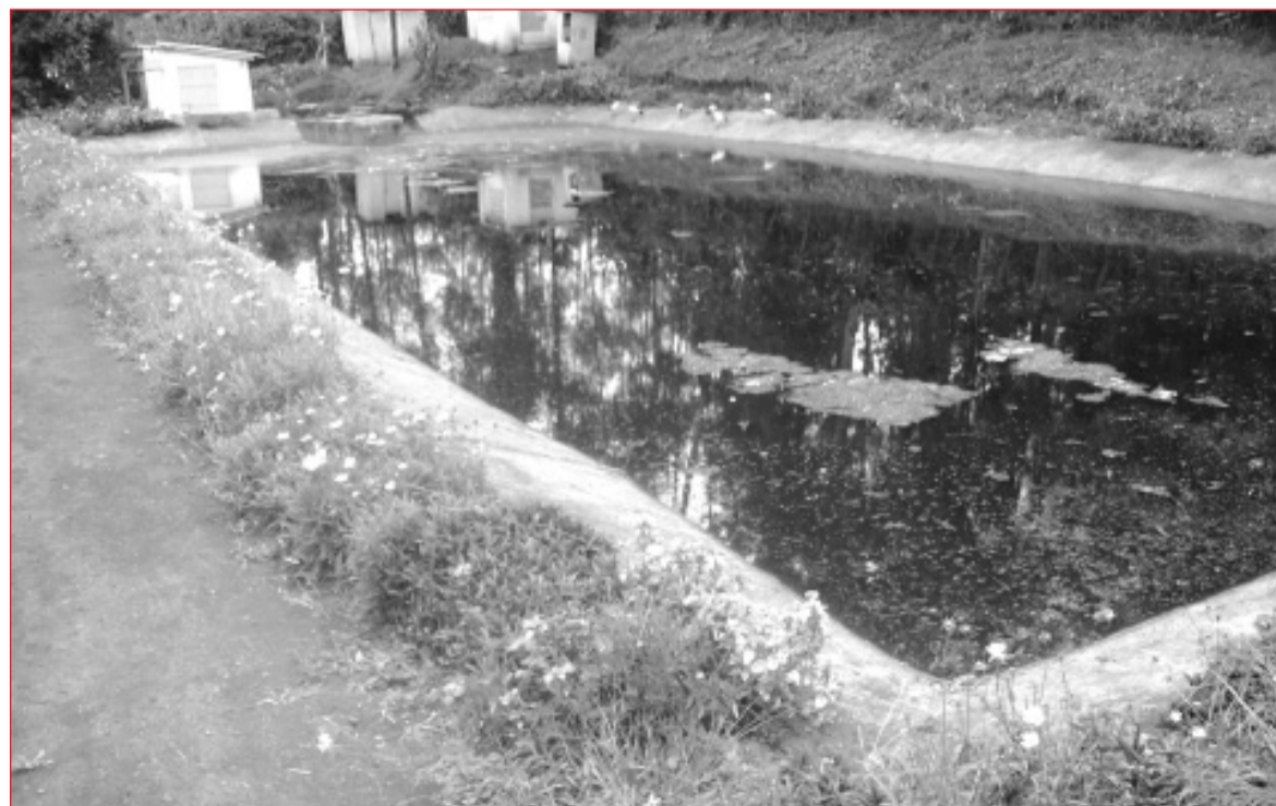
This is the sewerage system which is adjacent to River Kirigu in Karatina town.
