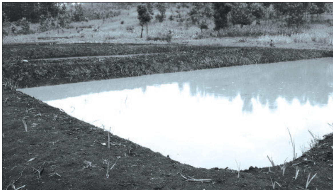
A fish pond constructed under ESP programme in Bungoma.
