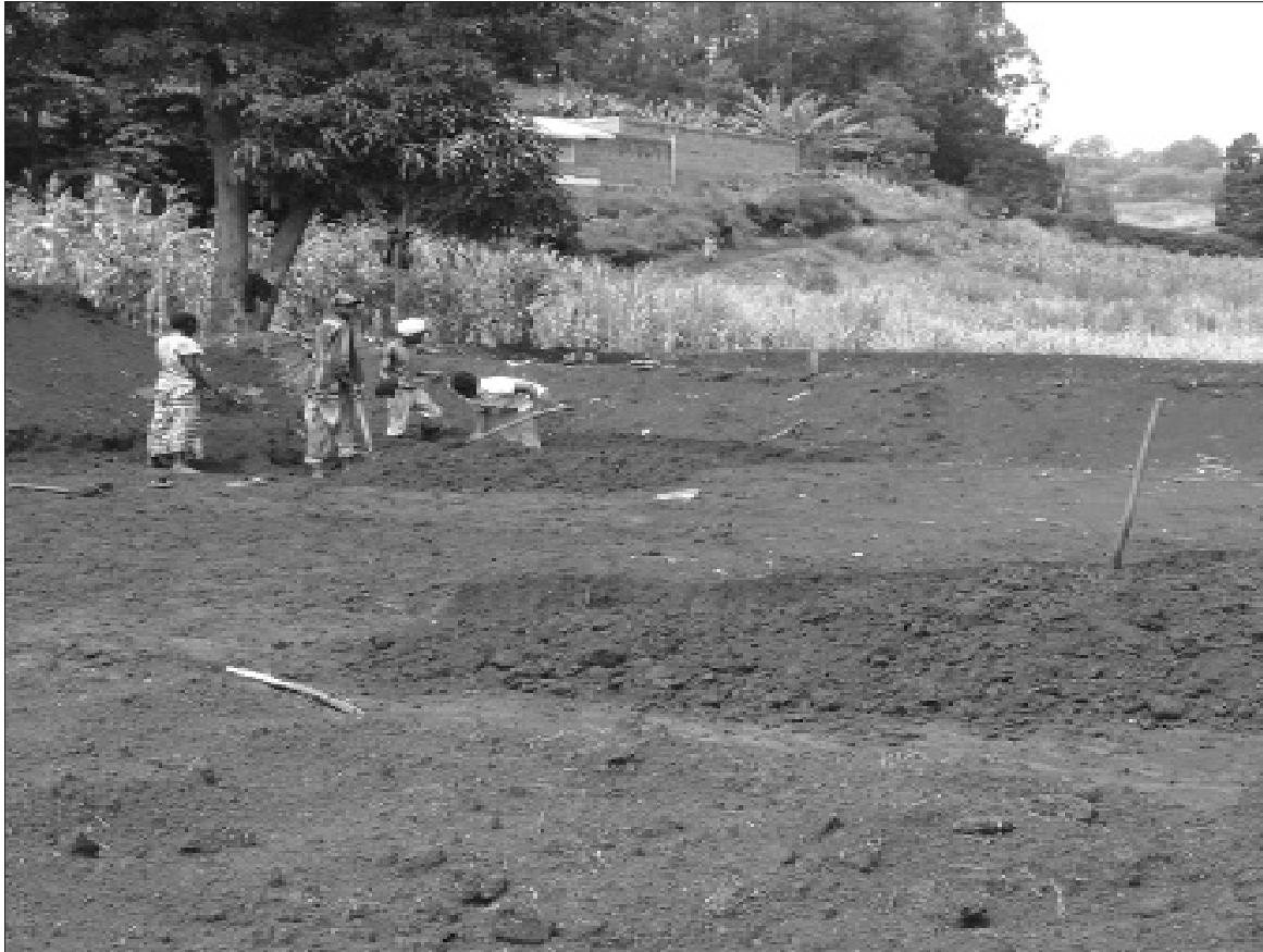
A Fish pond under construction.
