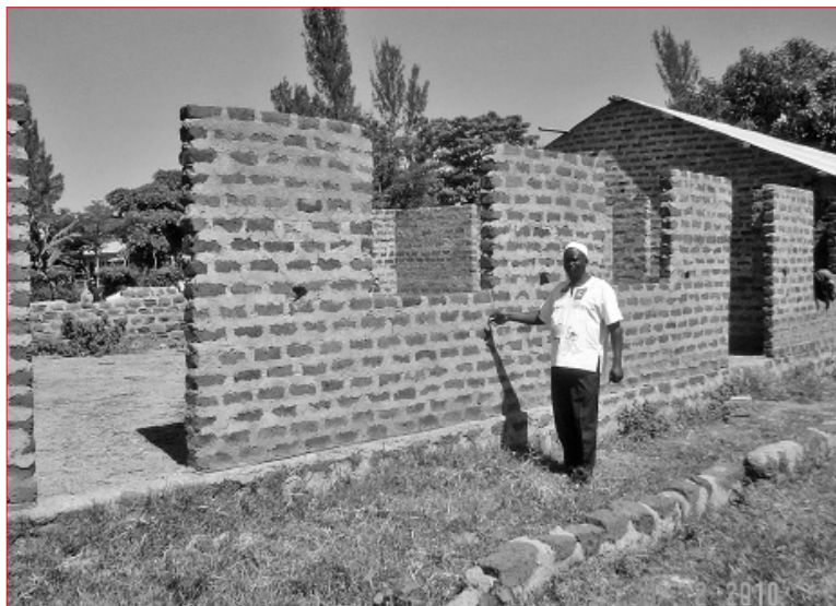
A school funded project under construction in Busia. Photo/Gilbert Ochieng
