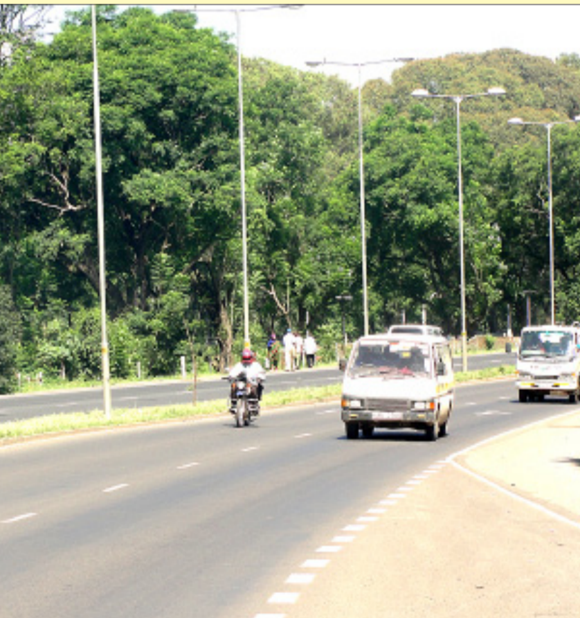
stretch of the Njoro-Lanet Highway. Photo/Fidelis Kabunyi
