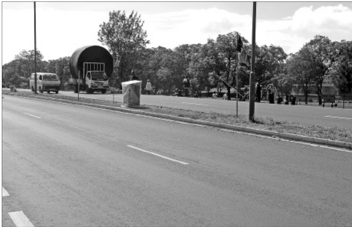
Road under construction. The region is set to embark on major infrastructural projects to enhance economic growth. Photo/File
