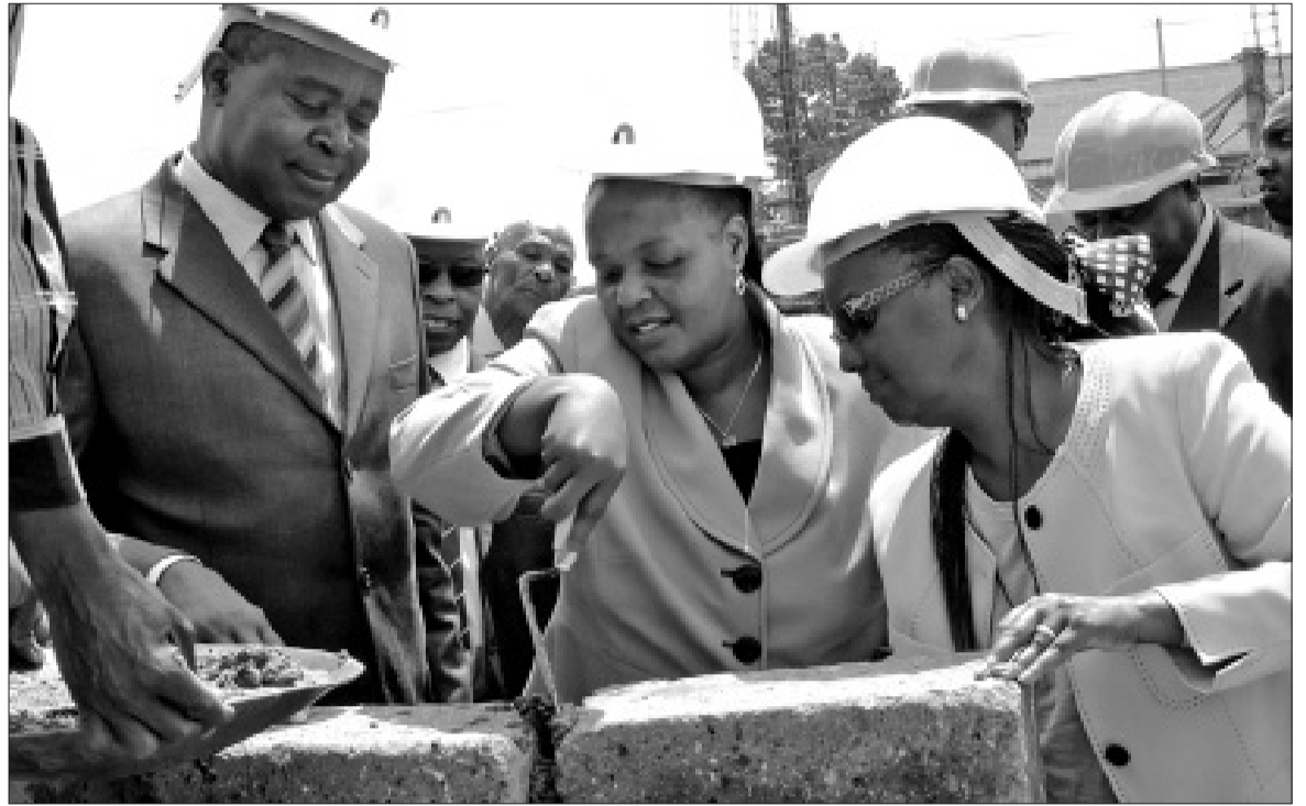
FROM RIGHT: Special Programmes Minister Hon. Esther Murugi, Housing Assistant Minister Margaret Wanjiru and Housing Minister Hon Soita Shitanda laying the foundation stone at Kamukunji traders market in Nyeri town recently. Photo/Joseph Mukubwa
