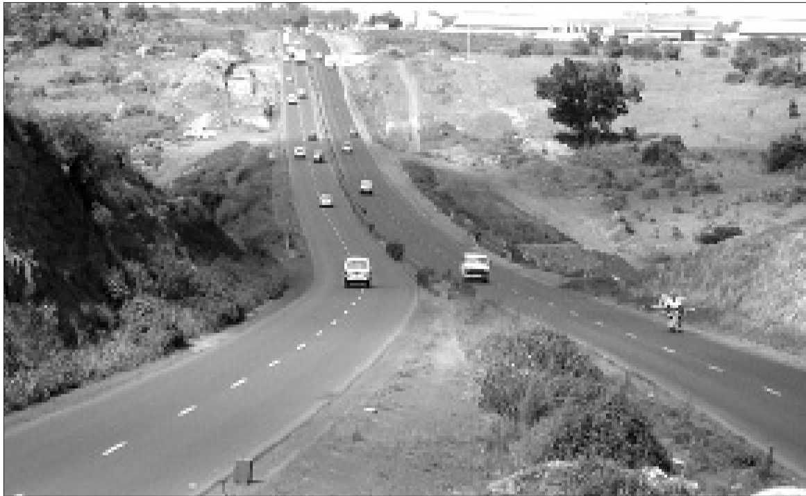
A section of finished road along Thika Road in Nairobi.
