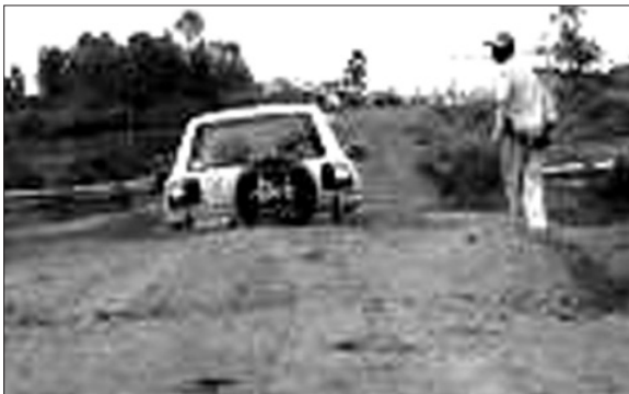
A vehicle going through a damaged road.
