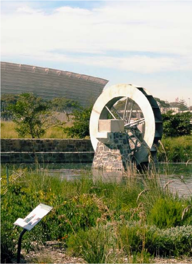
The new water wheel at Green Point Park set in motion by spring water piped from the Oranjezicht Springs. Energy generated from the wheel will be used to power lighting in the Park. Photo: Marijke Honig
