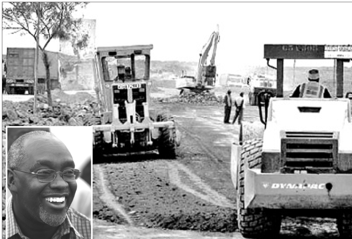
Road under construction. Inset: Mr. Franklin Bett, Roads Minister.
