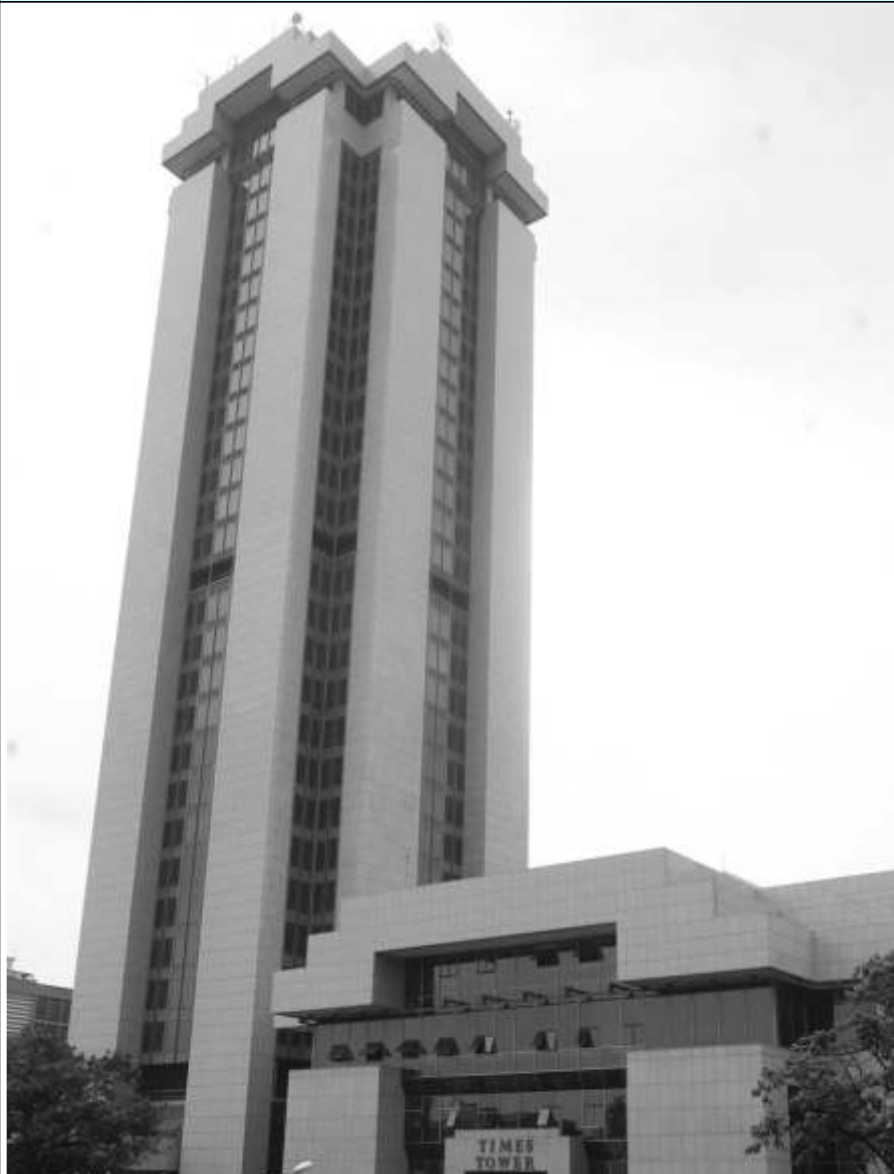
Kenya Revenue Authority headquarters in Nairobi.
