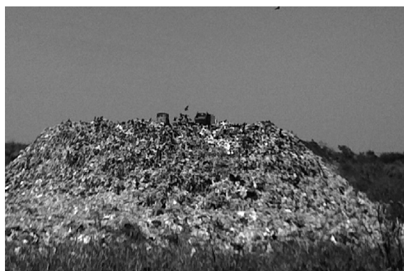
Picture 1; Rio Branco's Waste Disposal Site in 2005, notice the trucks on top of the waste mass.
