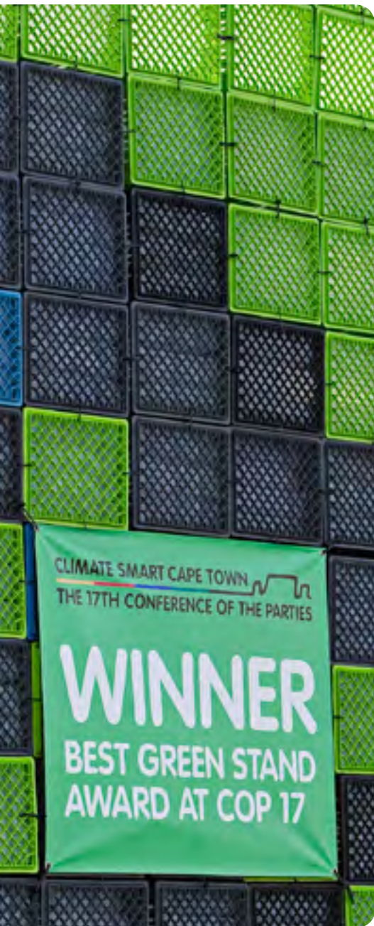
The Climate Smart Cape Town Pavilion, constructed out of recycled plastic milk crates, was awarded the best green stand award at COP17.
