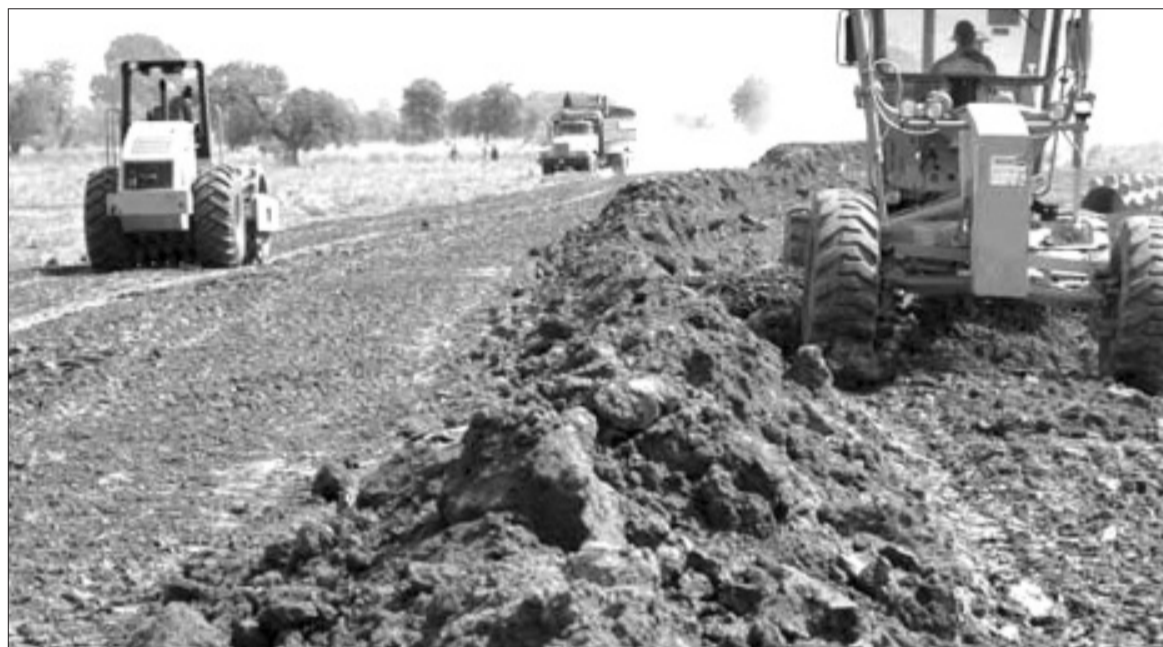
A section of the road under construction.
