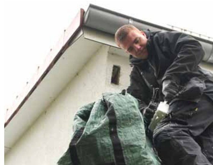
Steeplejack Benjamin Seider cuts the insulating block to size, fills in the gaps with grout, and the woodpecker's hole is sealed. But these repairs are not covered by insurance.
