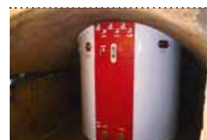
Wärme-Hamster, 4, hot water storage tank
