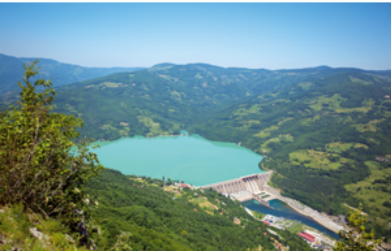
Dam on Perućac Lake on the border between Serbia and Bosnia-Herzegovina. A significant share (21.2 percent) of Serbia's energy supply comes from renewable sources.
