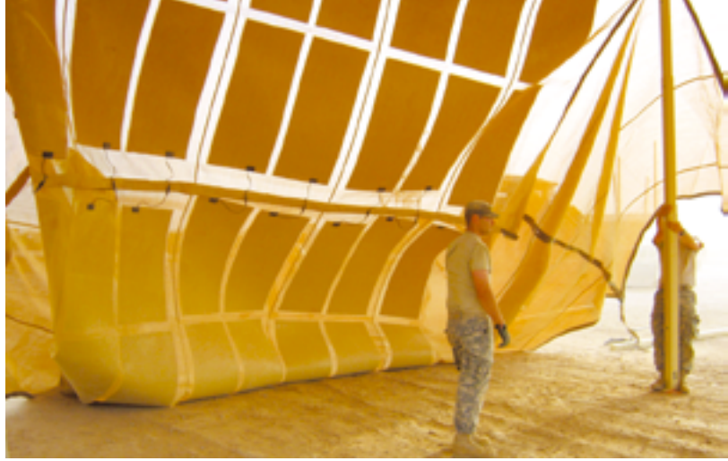
Flexible solar panels on US Army tarps at Camp Lemonnier in Djibouti. These enable the unit to generate the energy it needs to operate fans, radios and lighting.
