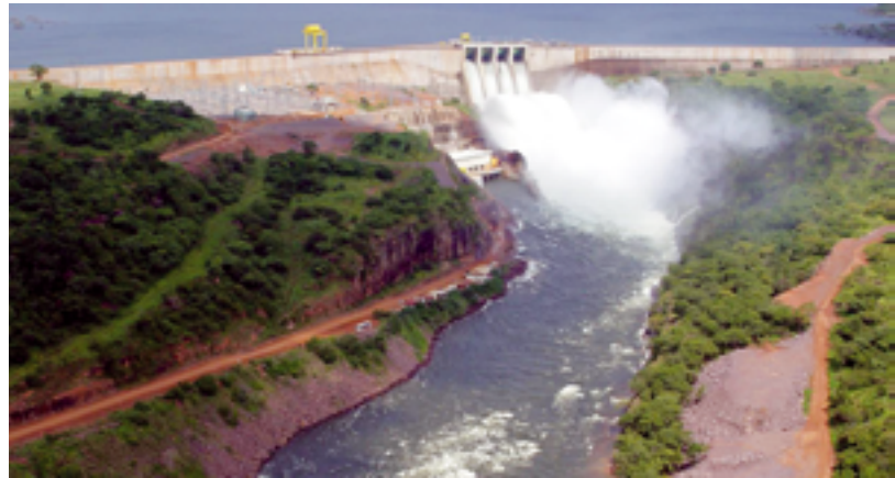
The Capanda dam on the Kwanza River in the Malanje province has four turbines that generate an output of 520 megawatts. The plant covers more than half of Angola's energy needs.
