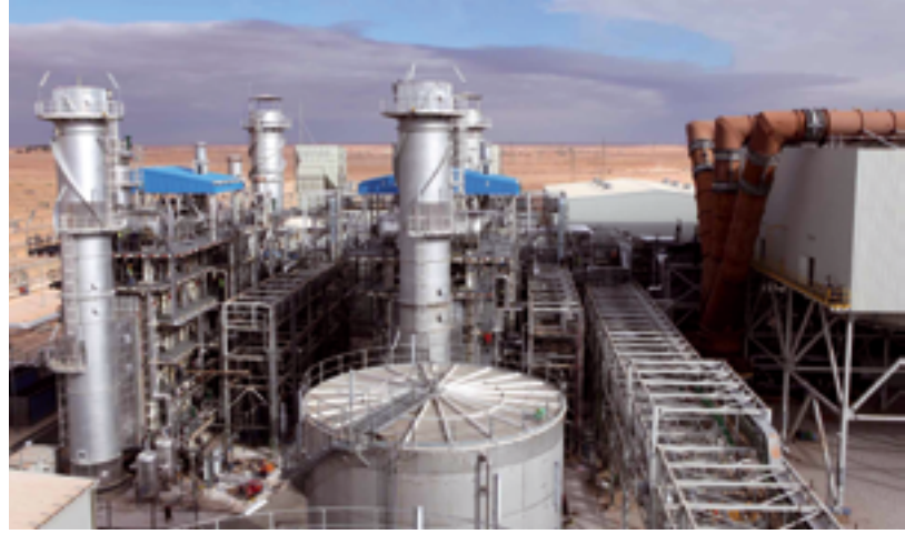
The Hassi R'Mel hybrid power plant in the Algerian province of Laghouat combines a solar thermal plant with a conventional combined cycle gas turbine.
