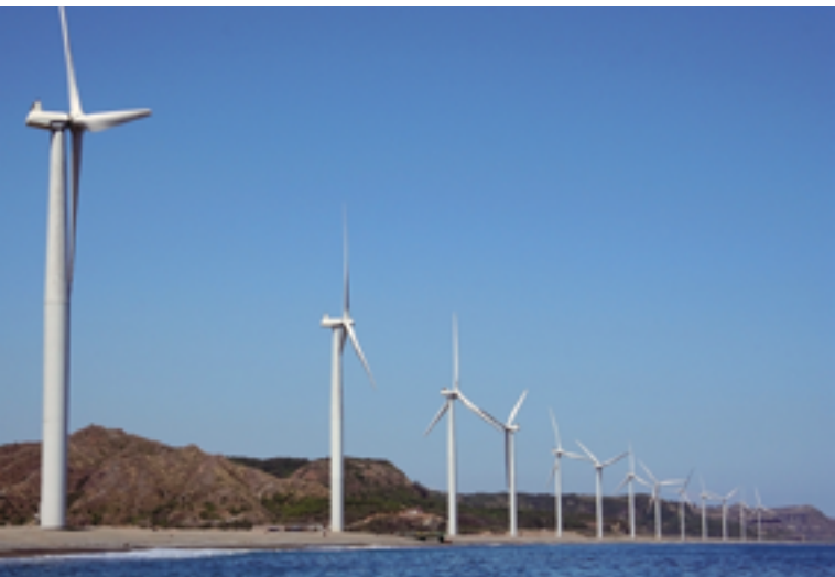
These wind turbines on the beach in Bangui, in the north of the island Luzon, were part of southeast Asia's first wind farm when they were inaugurated in 2005.
