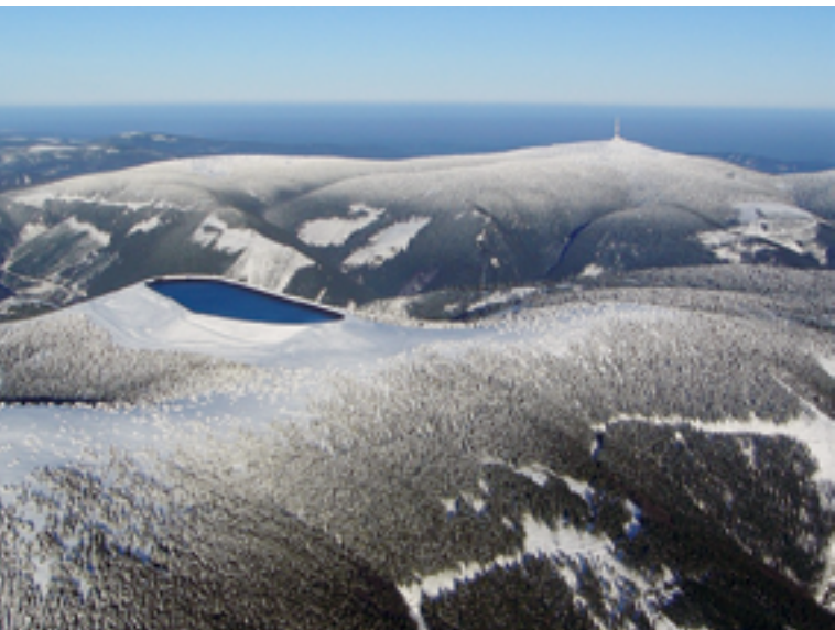
The Dlouhé stráně pumped storage plant is the largest of its kind in the Czech Republic, boasting a bottleneck output of 650 megawatts. The elevated reservoir is 1,350 metres above sea level.
