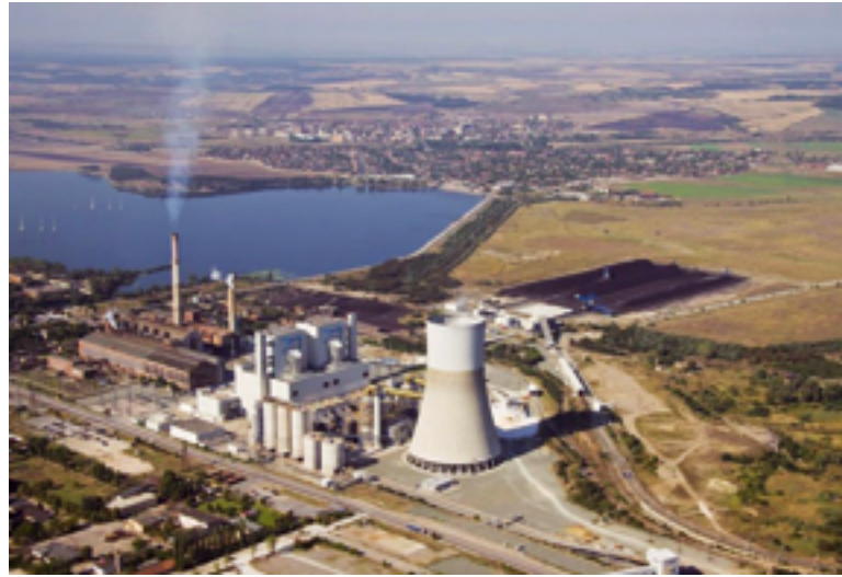
The coal-fired power plant in Galabovo in the Upper Thracian Plain is part of the Maritsa Iztok Complex, the largest energy complex in Southeast Europe. The lignite comes from the nearby open-cast mining area in the Sakar Mountains.
