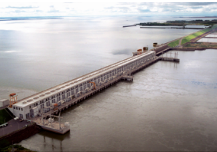
Equipped with 20 turbines, the Yacyretá dam on the Paraná River at the border between Paraguay and Argentina supplies around a quarter of Argentina's electricity needs.
