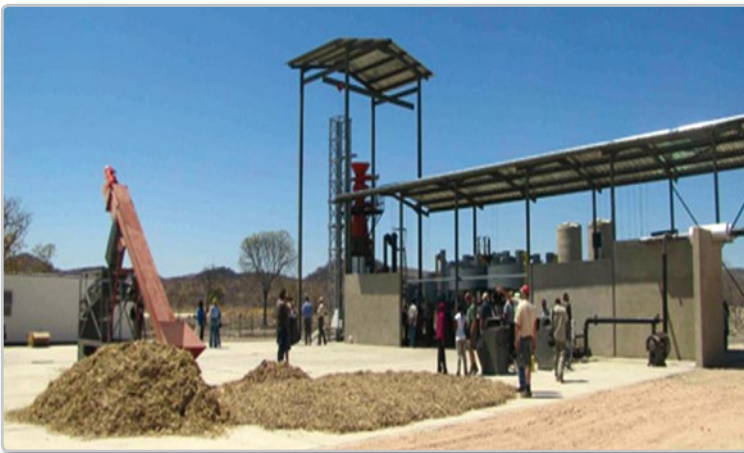
Figure 46: Namibia's first IPP, a biomass-powered pilot plant of 250 kW, farm Pierre [71]
