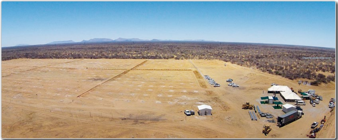
Figure 47: Preparations for InnoSun's Omburu solar power station close to Omaruru [73]
