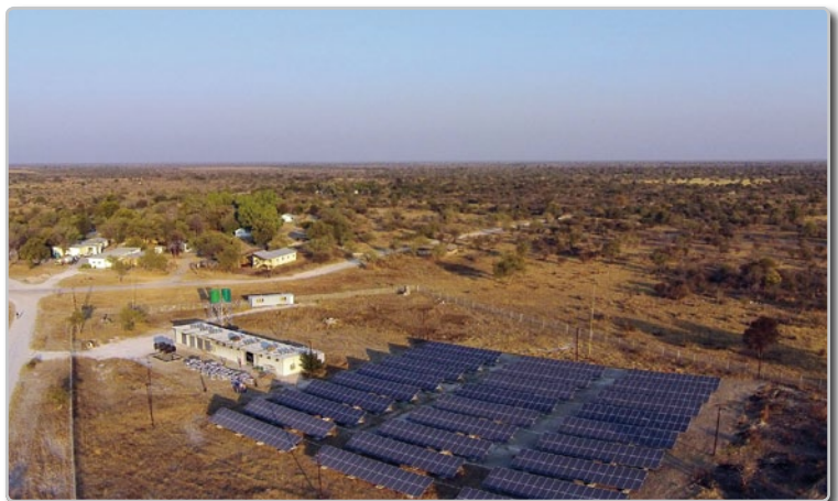
Figure 16: The diesel-solar PV hybrid powering the off-grid community at Tsumkwe [26]
