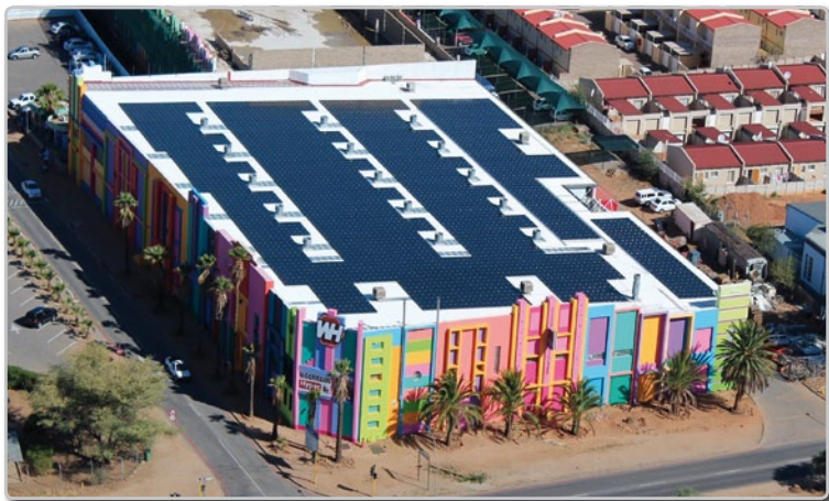
Figure 33: Commercial grid-connected solar photovoltaic plant powering Woermann Group Supermarket, Windhoek [50]
