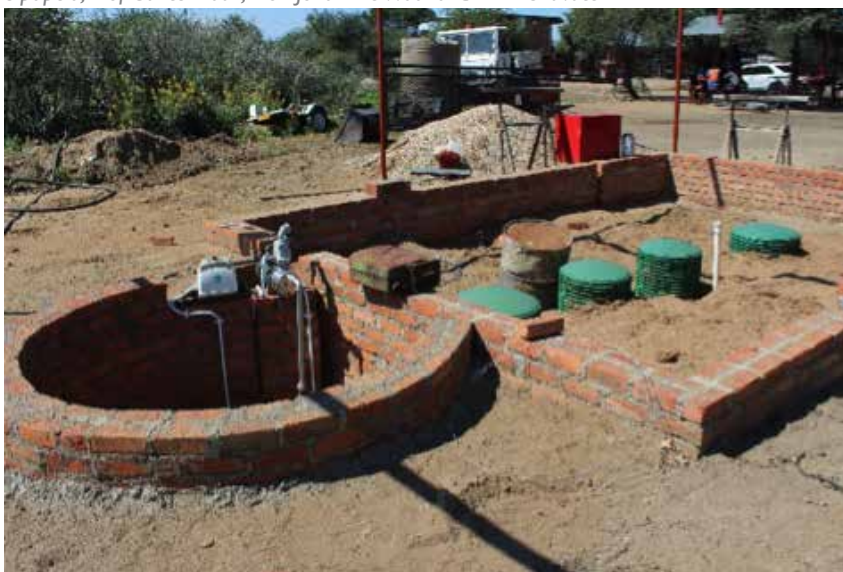
Jumbo Charcoal's water recycling plant - water from kitchen and shower-baths recycled for use to watering garden.
