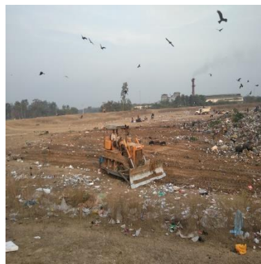
Leveling of dump site
