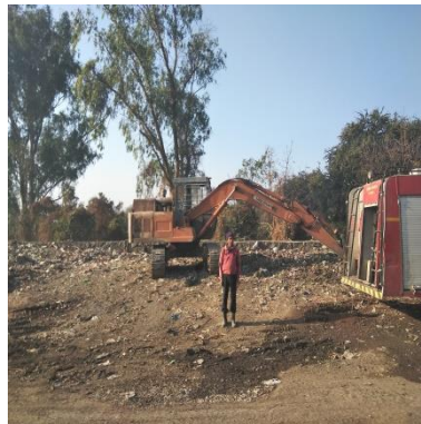
Equipments for compacting
