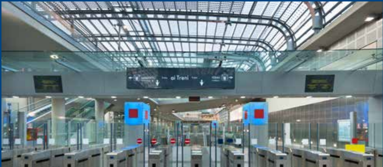
The glazing of the railway station Porta Susa Torino is equipped with mono-crystalline photovoltaic cells. Besides generating electricity, they also act as a sun shield. Source: © Dario Egidi, iStockPhoto
