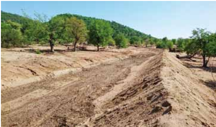
Diversion drain within Nyanyadzi catchment
