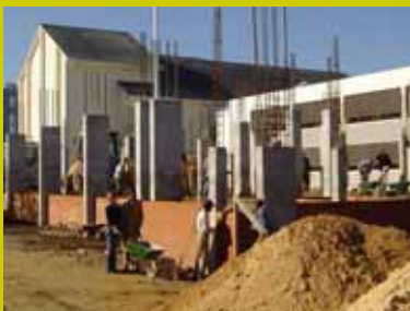
The Green Building's first phase, June 2004
