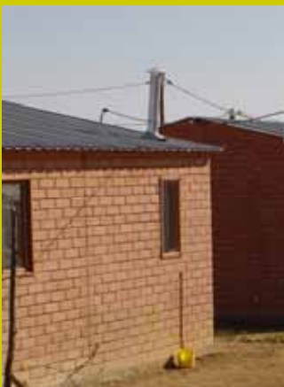
An installed chimney in Kathrada Square
