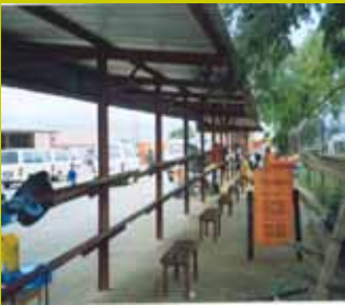
The new structures of the vendors' stalls.(Ngobeni & Machumele,2004)
