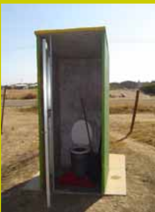
An installed VIP that replaced the bucket system
