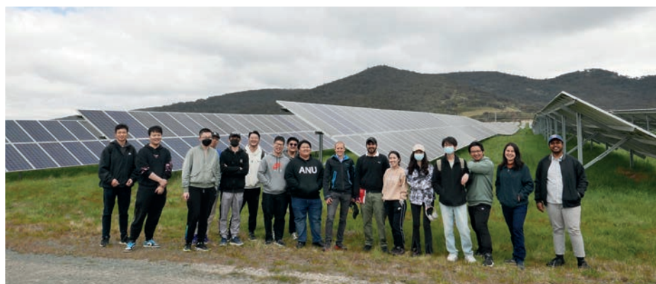
Royalla Solar Farm
