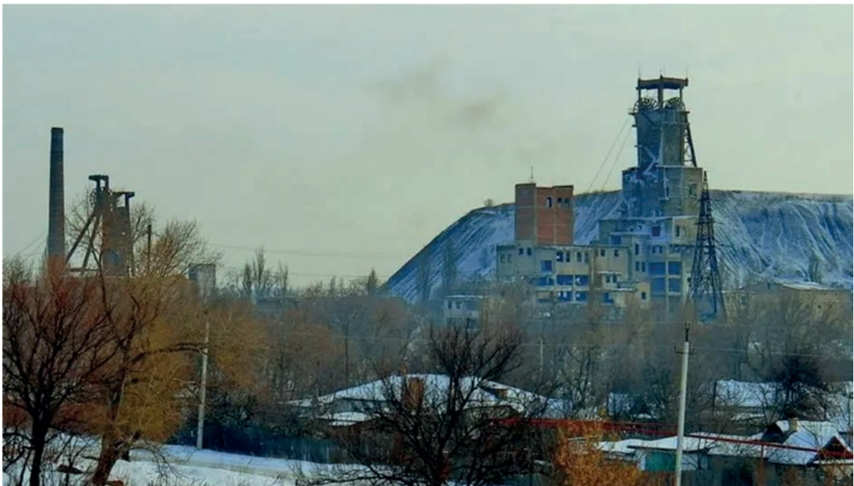
Photo 8. In March 2018, the occupation "Ministry of Coal and Energy of the DPR" announced the cessation of water pumping at the Yuny Kommunar mine
