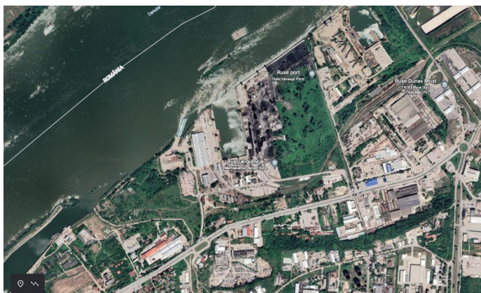
Figure 6 Port Ruse East-general view, Google Earth
