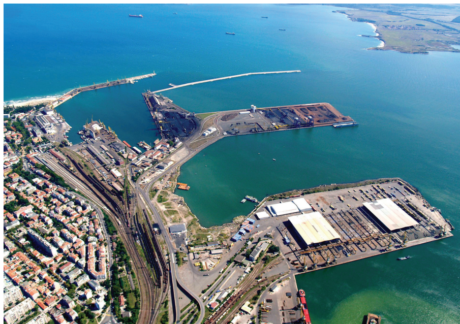
Figure 12 Port Burgas-general view
