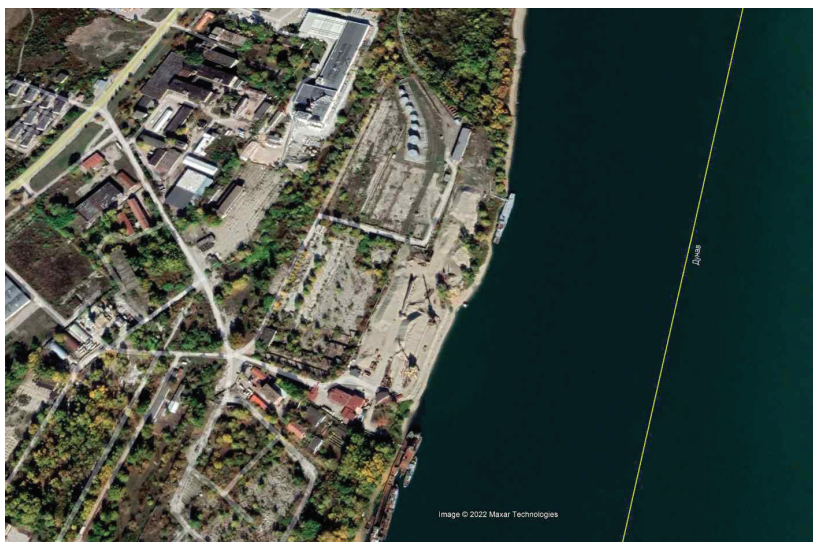
Figure 9 Port terminal Vidin South - general view, Google Earth
