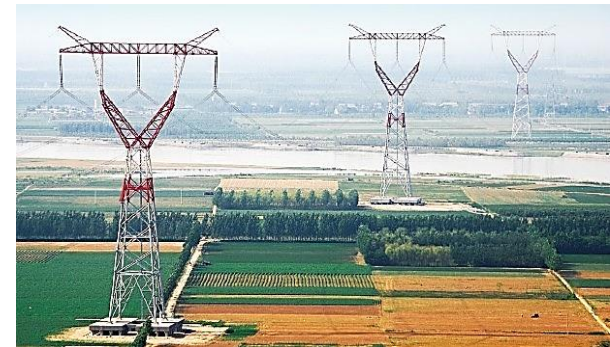
Jindongnan to Nanyang to Jingmen 1000kV UHV
