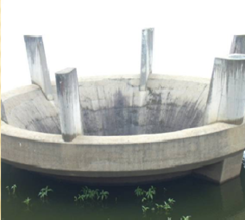
Picture n°7: Damming level in 2004
