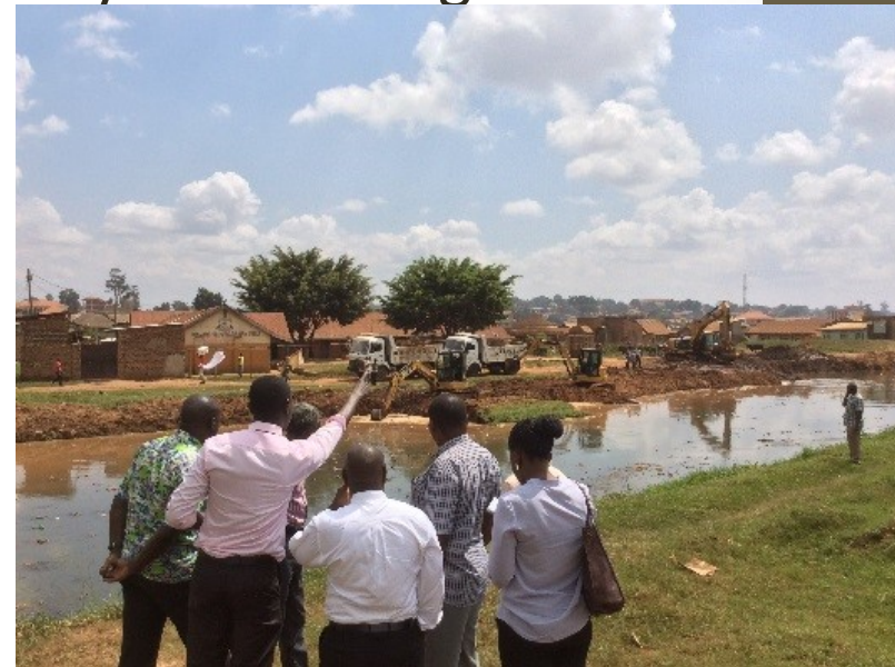
desilting of drainage channel at Bwaise, Kampala
