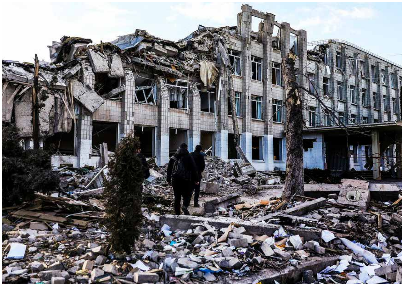
The destroyed main building of a school in Zhytomyr, Ukraine.
