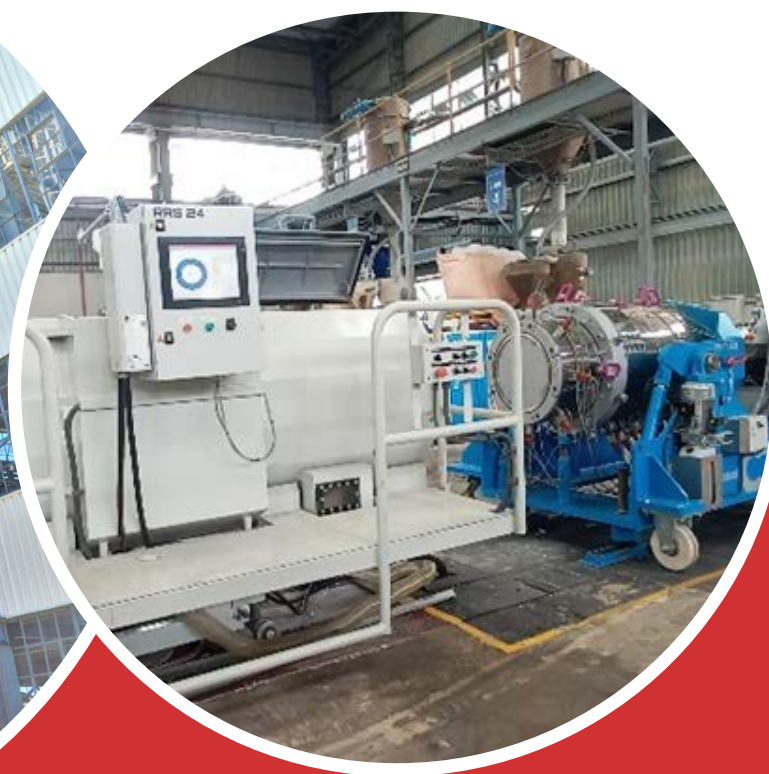
Proplastics New Mixing Plant Silos
