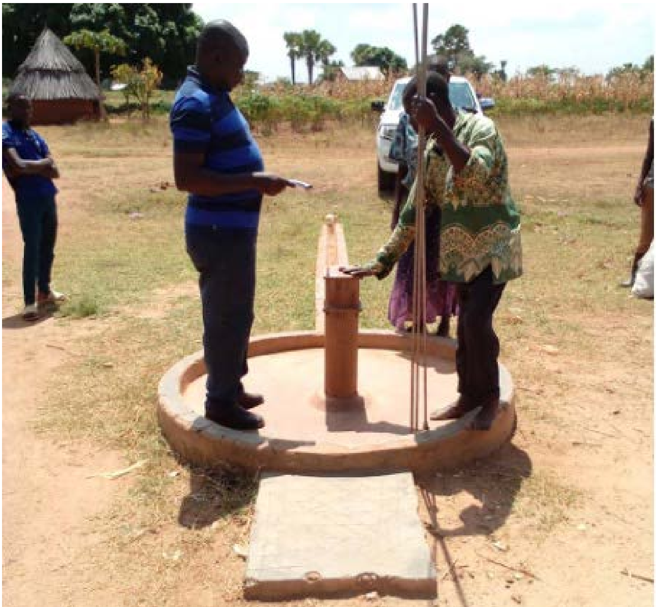
A borehole in Akonye bedo Sub County in Gulu district being assessed; Pending rehabilitation.
