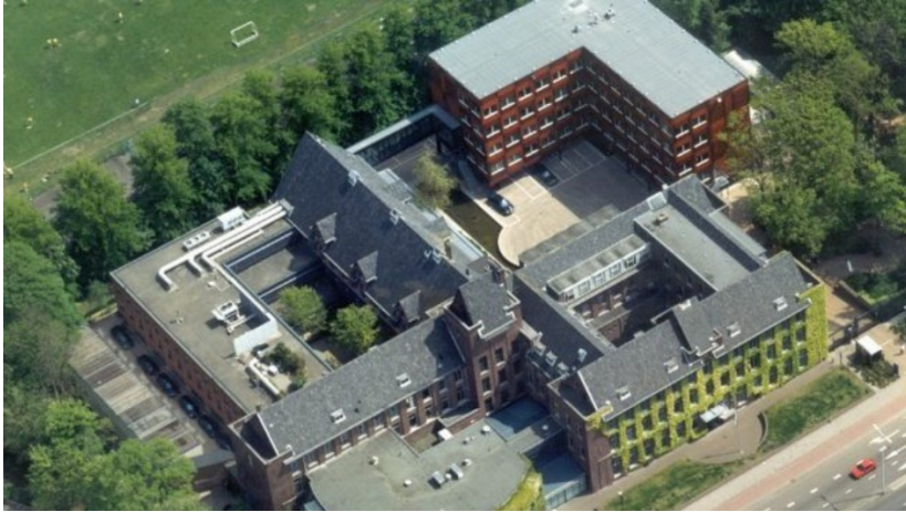
The Specialist Chambers building in The Hague. Photo: Europol.
