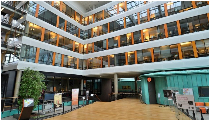
Council of Europe's "Agora" building in Strasbourg. Photo: Wikimedia Commons/Adrian Grycuk
