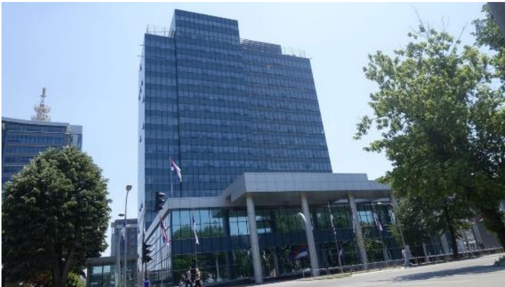
The RS Government building, Photo: EPA/Mikko Pihavaara.
