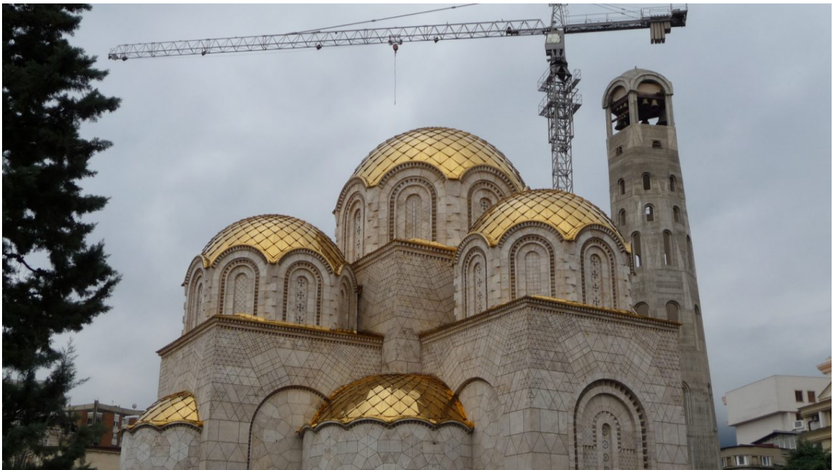
For a long time the construction was backed politically but shrouded in secrecy. Photo: BIRN
