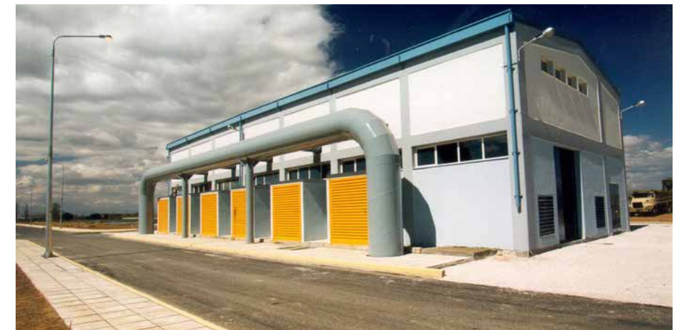
Figure 3-51 Thessaloniki's WWTP is equipped with 5 aeration units
