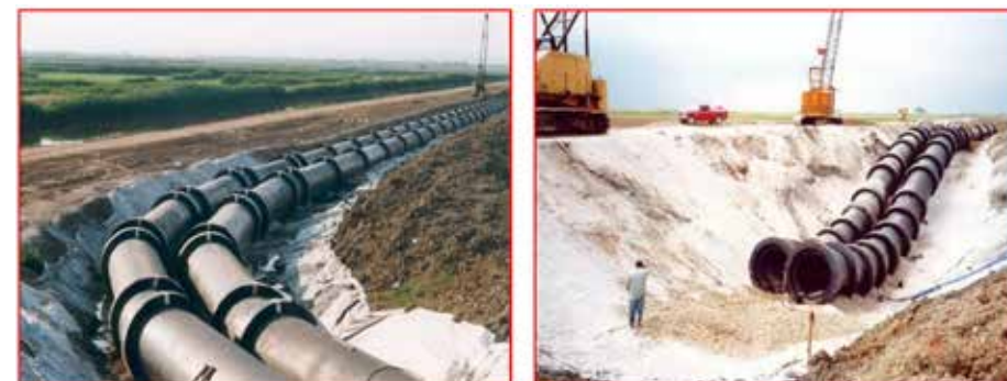
Figure 3-56 Treated wastewater disposal to Thermaikos bay, through submarine outfalls
