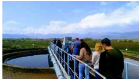
Figure 6-9 Visit in Florina's Waste Water Treatment plant (April 2018)
