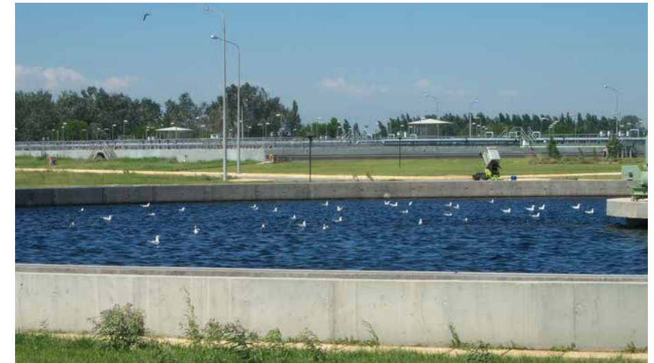
Figure 3-48 Primary sedimentation tanks in Thessaloniki's WWTP
