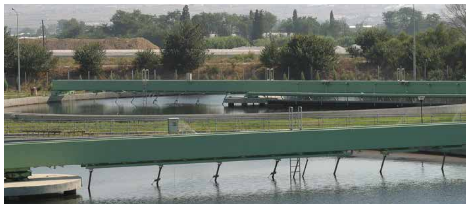
Figure 3-47 Stormwater tanks in Thessaloniki's WWTP
