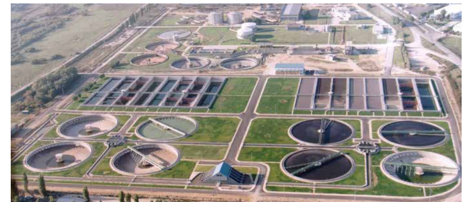
Figure 3-42 Aerial photo of Thessaloniki's main WWTP (Sindos)
