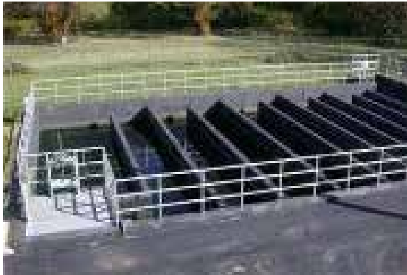
Figure 3-53 Disinfection of treated wastewater with chlorination
