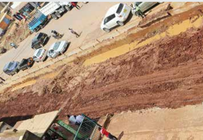
Ongoing construction of drainage systems and service lane in Mbale town
