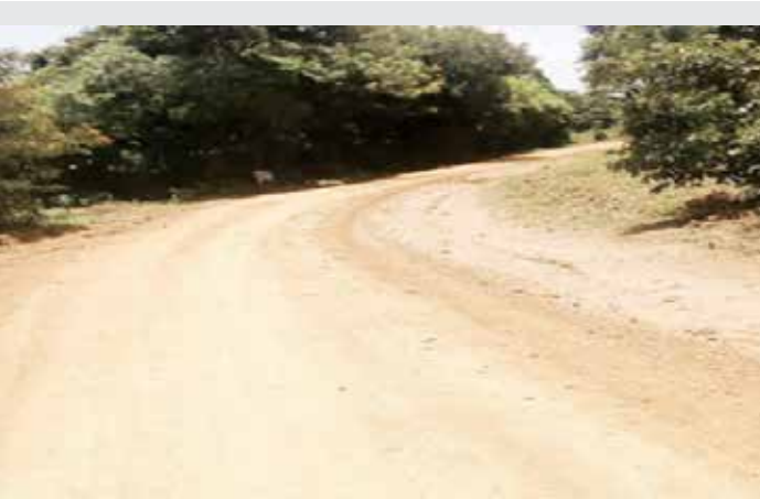
Upgraded murrum road within Siaya County
