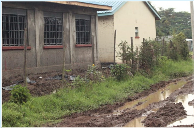
The state of the road next to the Health Centre, along River Auji
